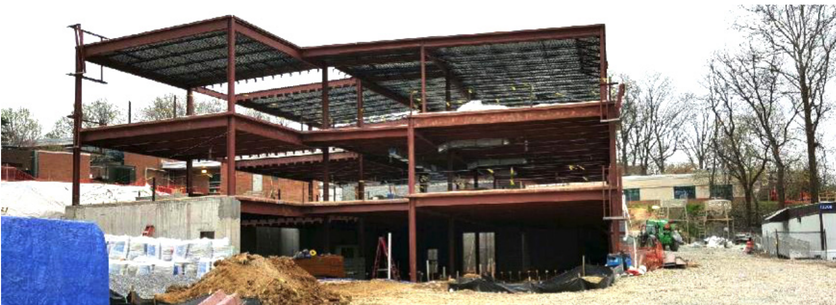
Construction of the Three-Story Addition at McKinley Elementary School
