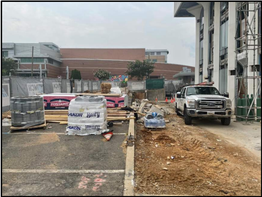
View of New Ramp Area to Washington Liberty High School
