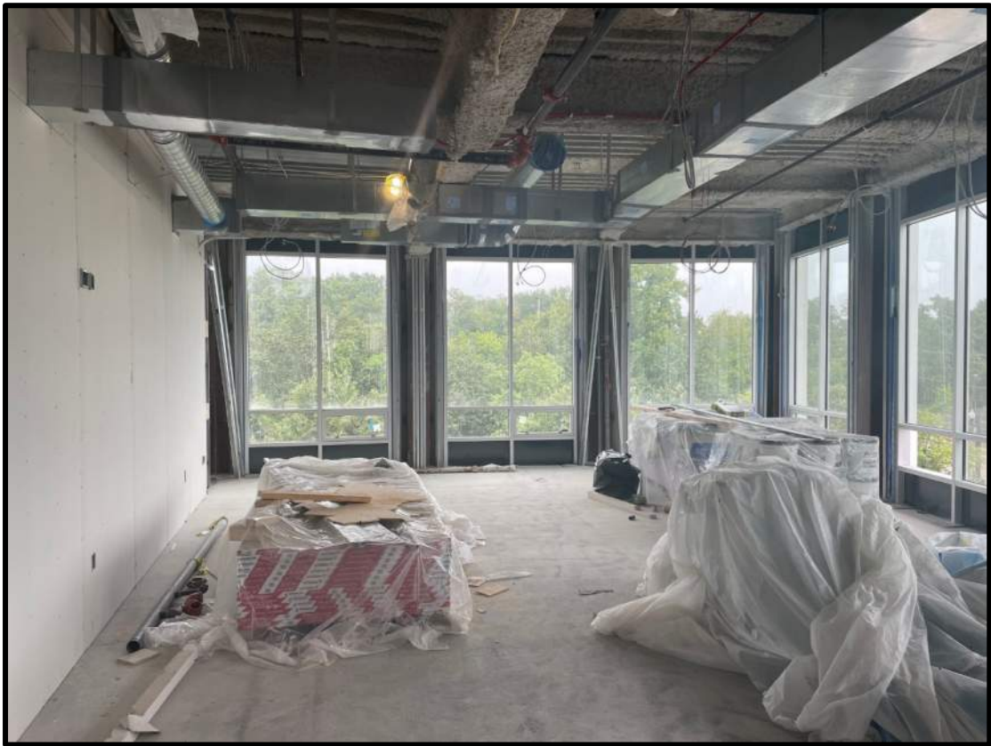
View of Work Ongoing on Level 2
