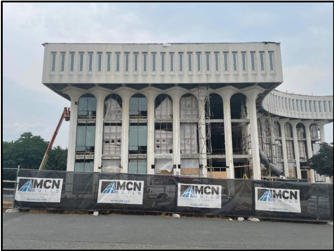
View of the Building from Washington Liberty High School
