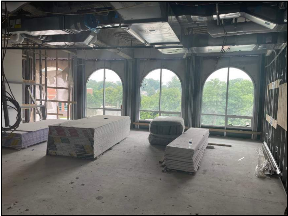
View of Work Ongoing on Level 3
