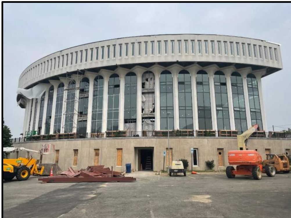
View of the Rear of the Building
