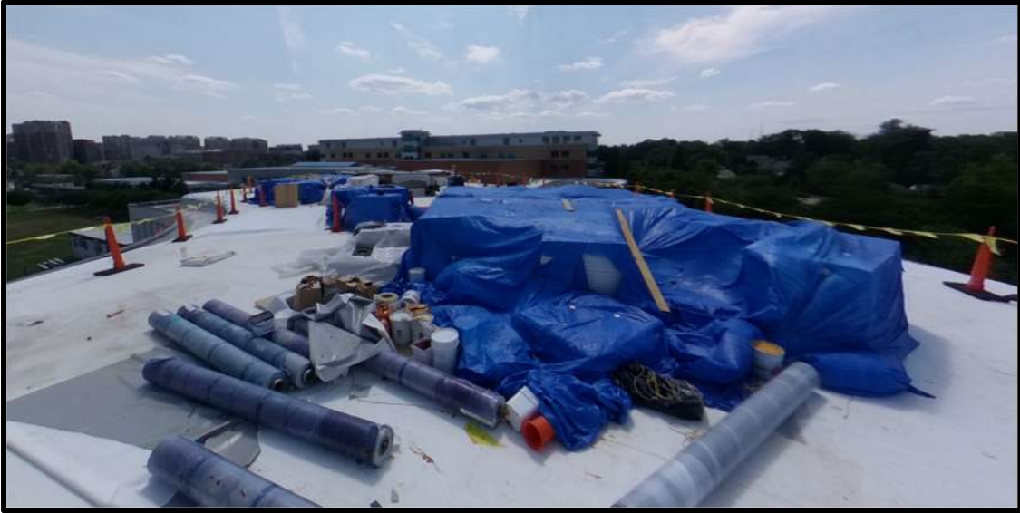
View of Working Ongoing on Roof
