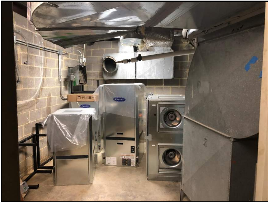
View of Working Ongoing in Planetarium
