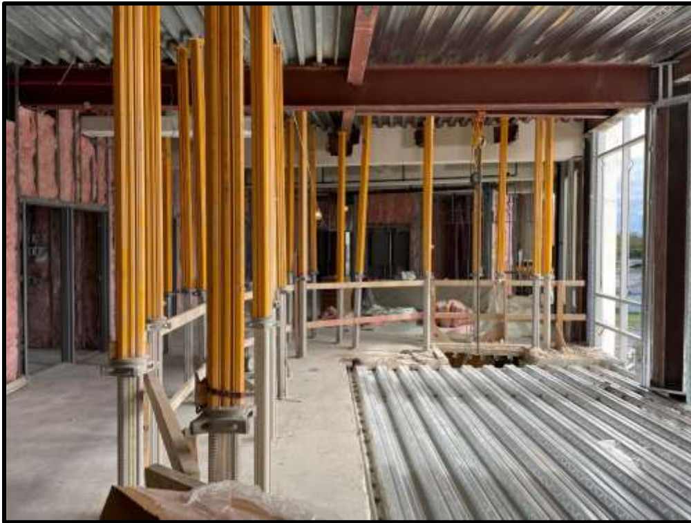
View of Work Ongoing on Level 2
