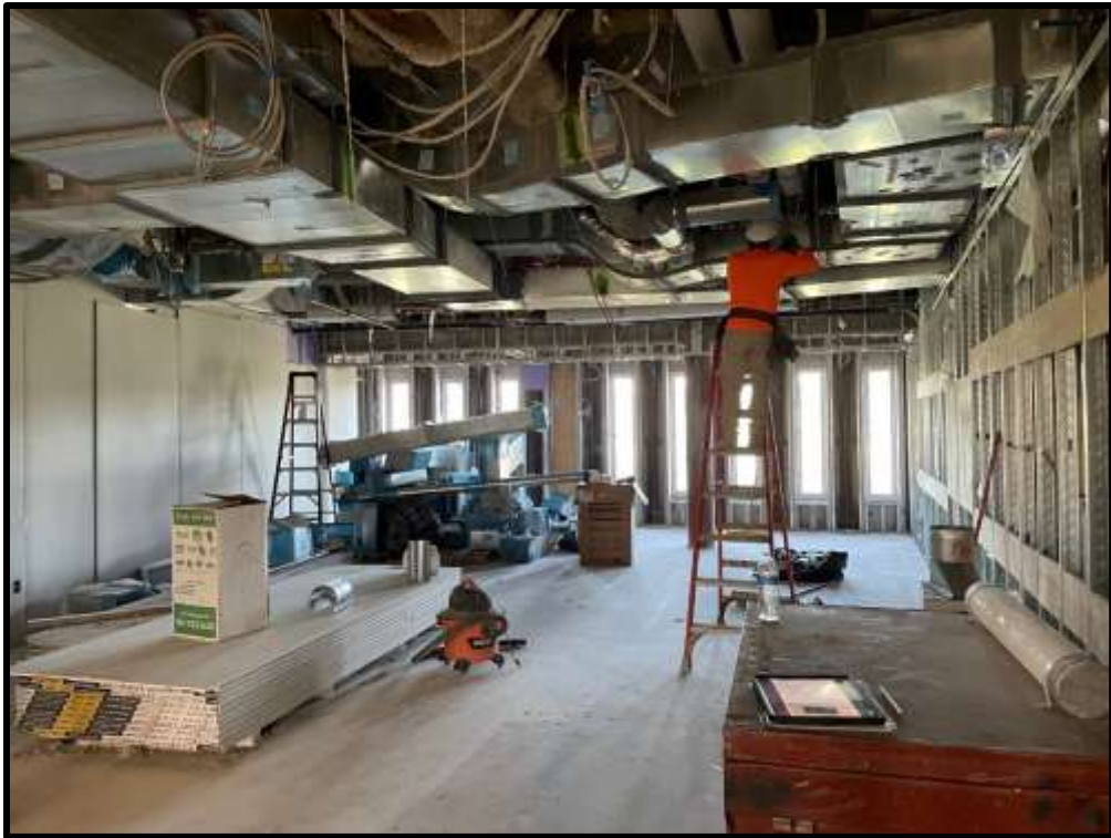
View of Work Ongoing on Level 4
