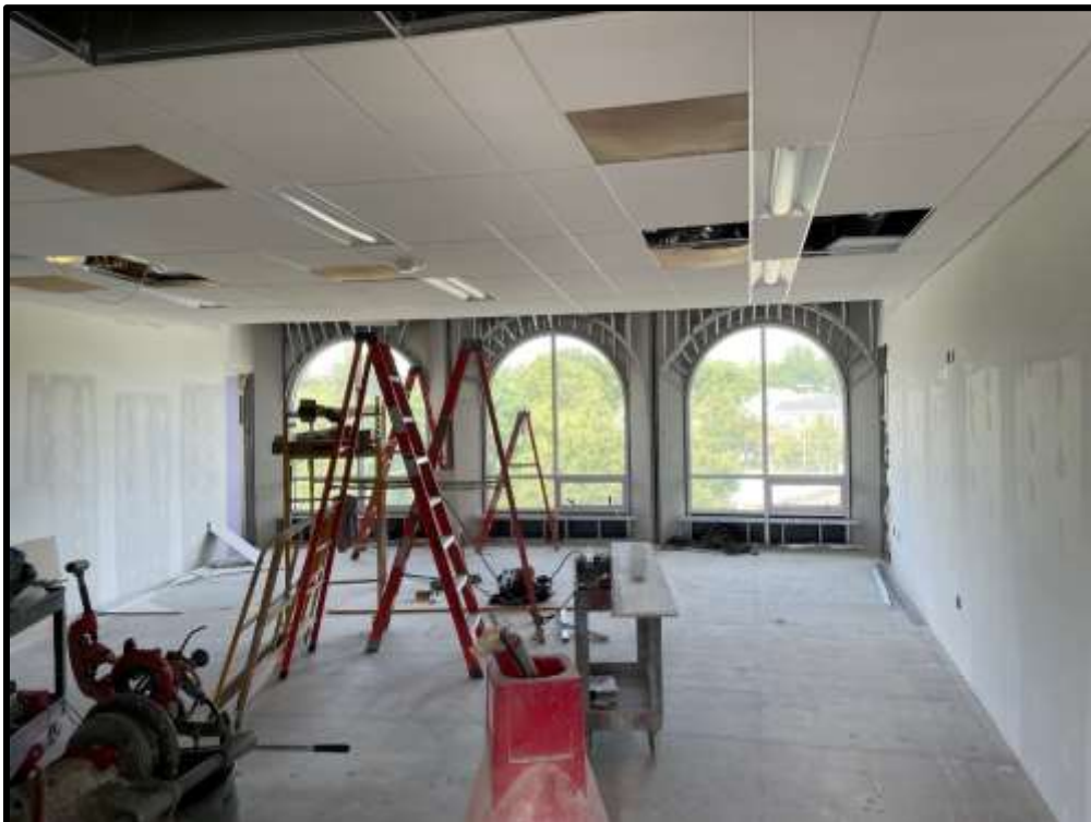
View of Work Ongoing on Level 3
