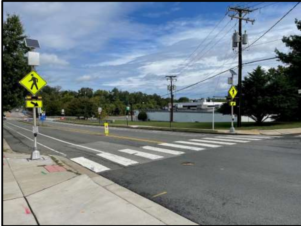
View of Finished RRFBs Along North Quincy Street
