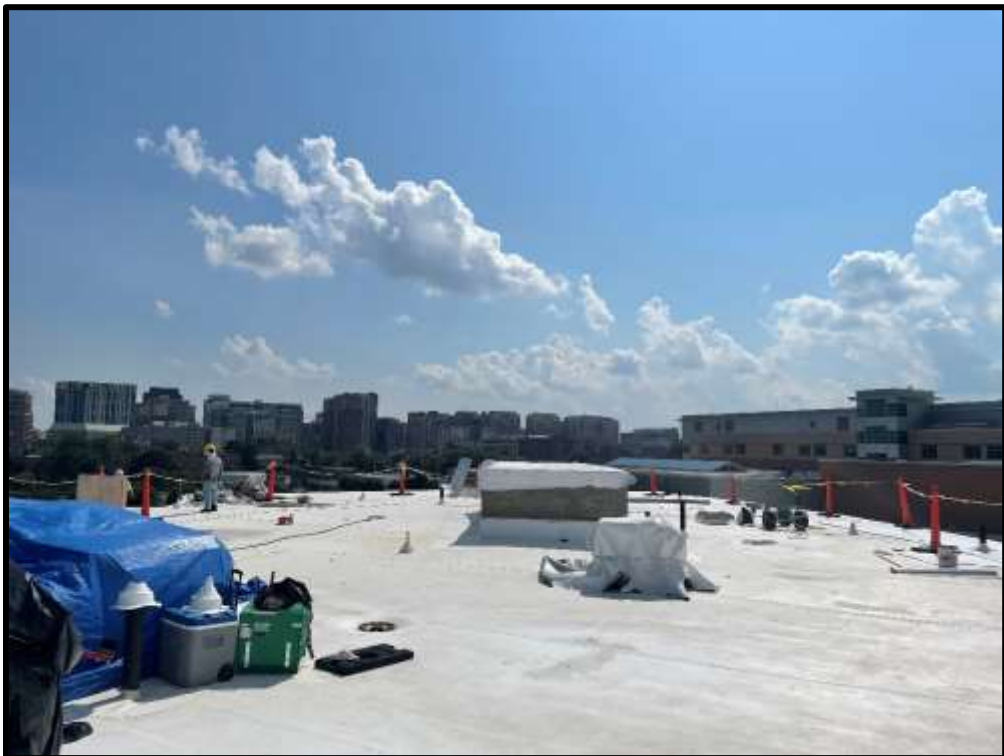
View of Working Ongoing on Roof
