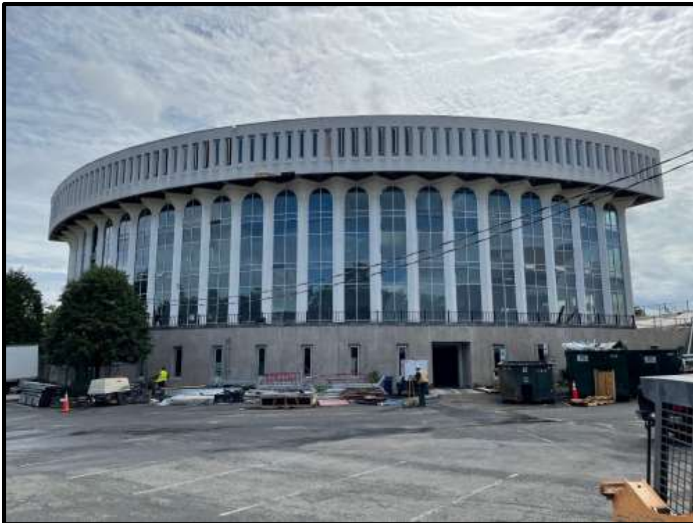
View of the Rear of the Building
