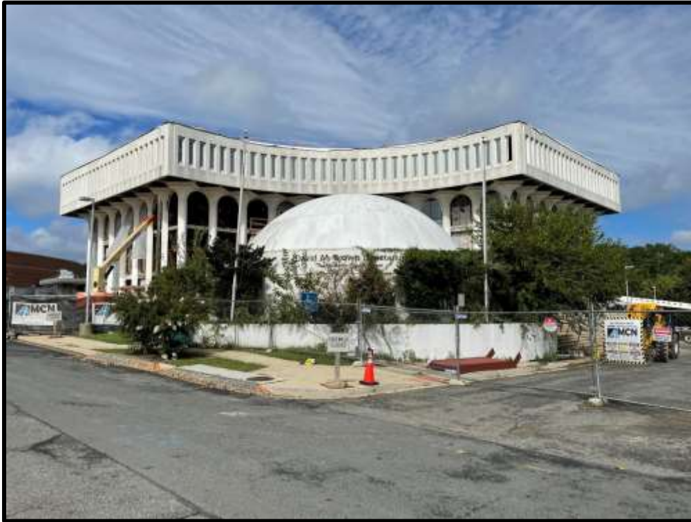
View of the Front of the Building
