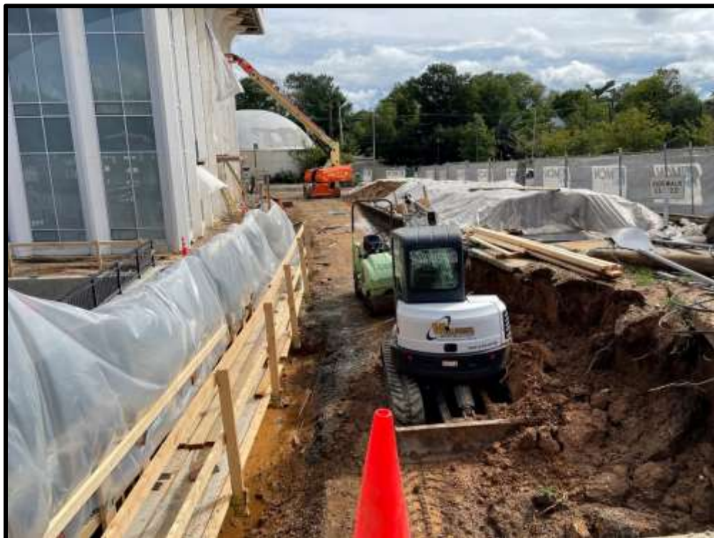
View of Work Ongoing on Ramp to Washington Liberty High School
