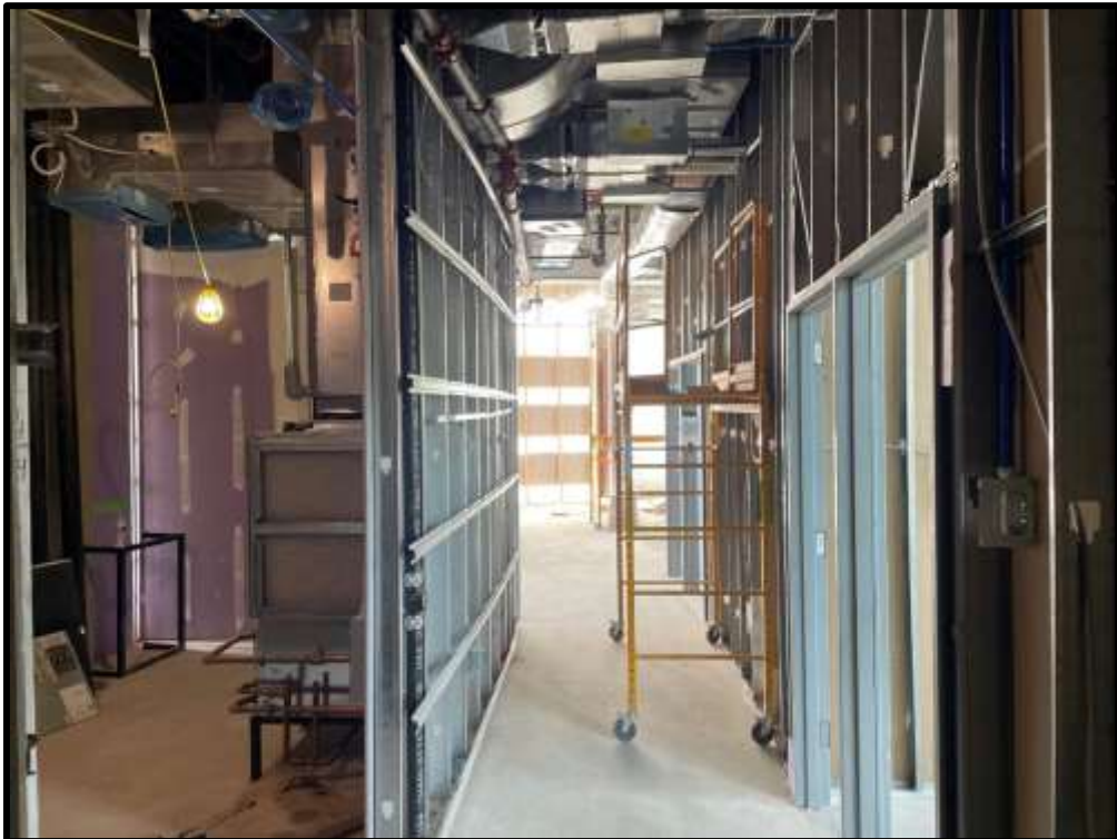
View of Work Ongoing on Level 1
