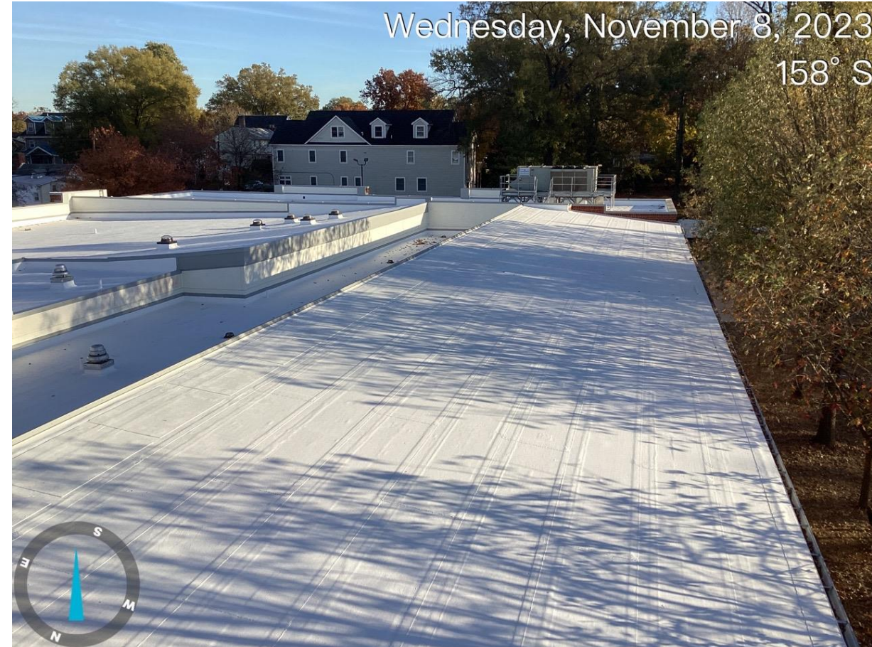
Randolph Roof Replacement Project Fall 2023
