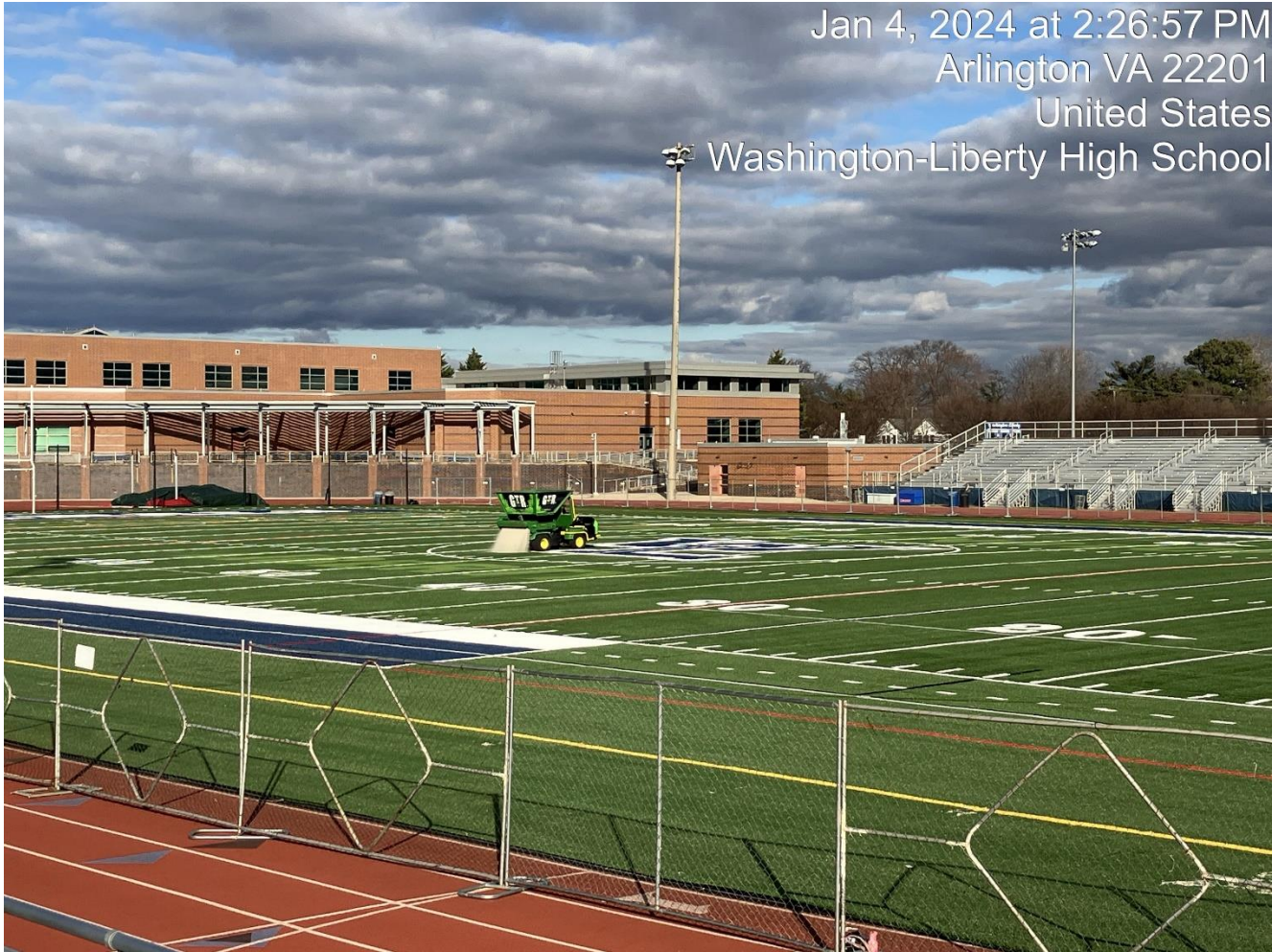
Washington-Liberty Synthetic Turf Replacement Project Early Winter 2024
