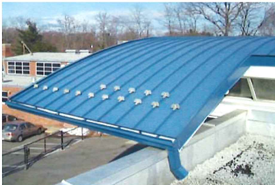
Photo 4: Barrel roof standing seam minor missing snowguards on Area N.
