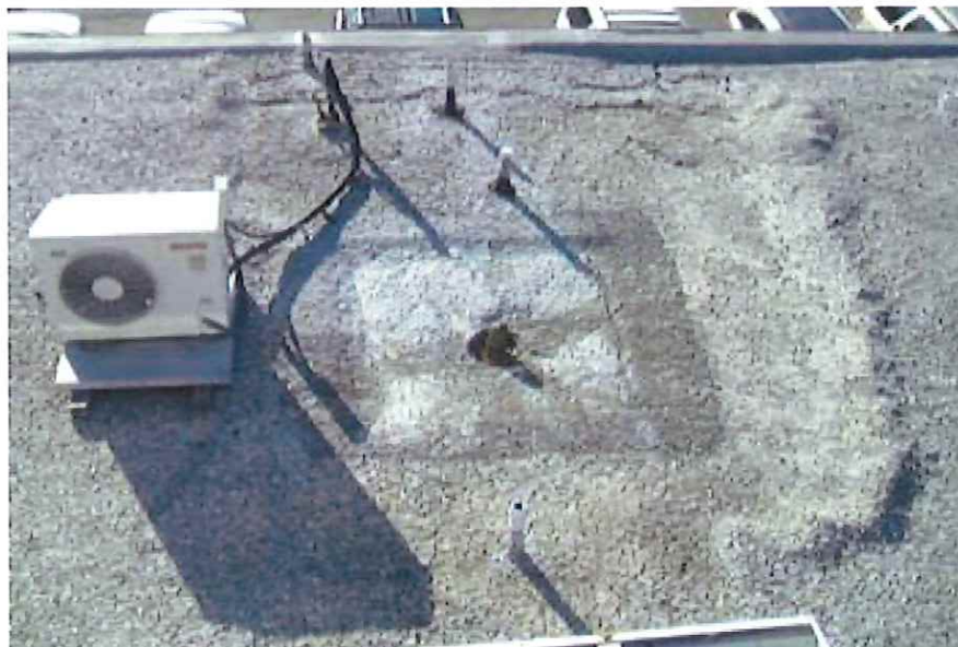
Photo 2: Extensive roof drain repair work on Area F
